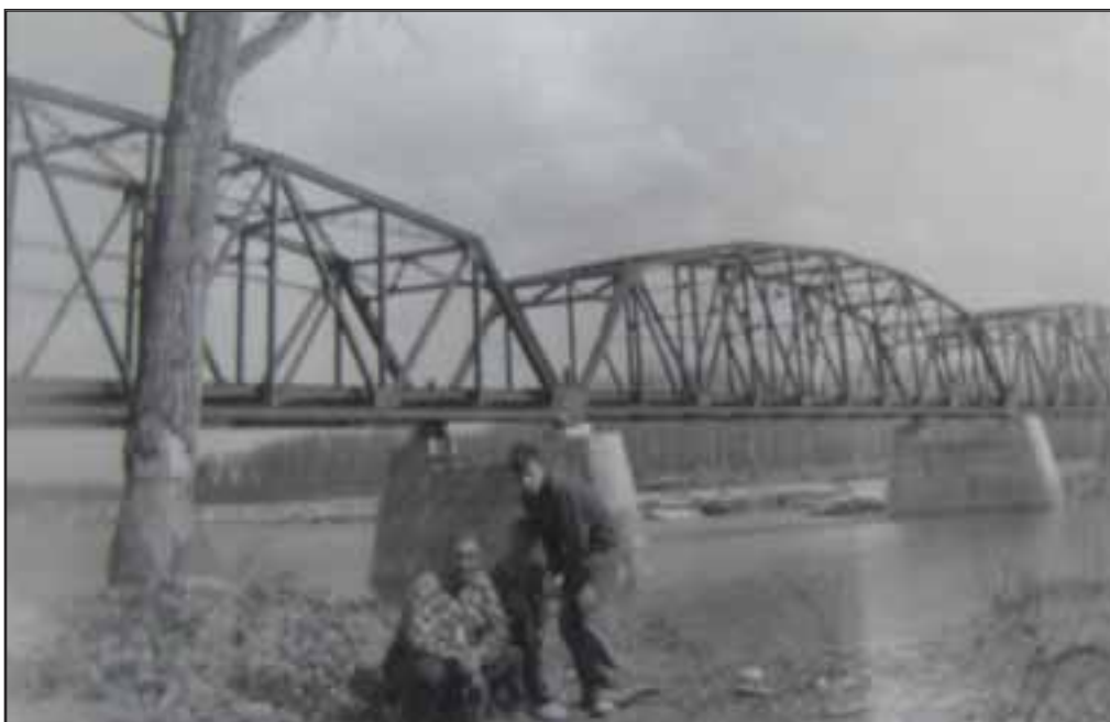
On March 27, 1954 residents of Fort Assiniboine were thrilled at the announcement that a 'bridge would be built leading into the community of Fort Assiniboine. On Aug. 15, 1956 the bridge was officially opened with approx. 4000 attendees who came to celebrate the completion of the bridge.
