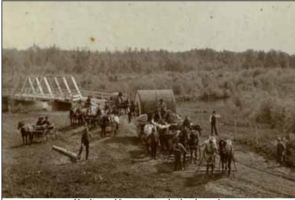
Hauling a 10 ton marine boiler down the Athabasca Landing Trail, late 1800s/early 1900s.
